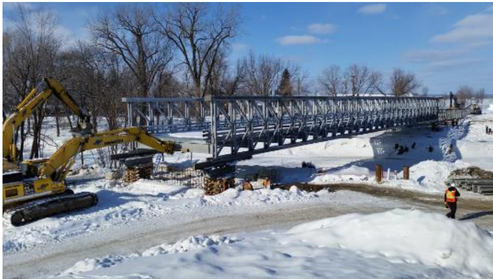
Figure 7: Modular Panel Bridge
