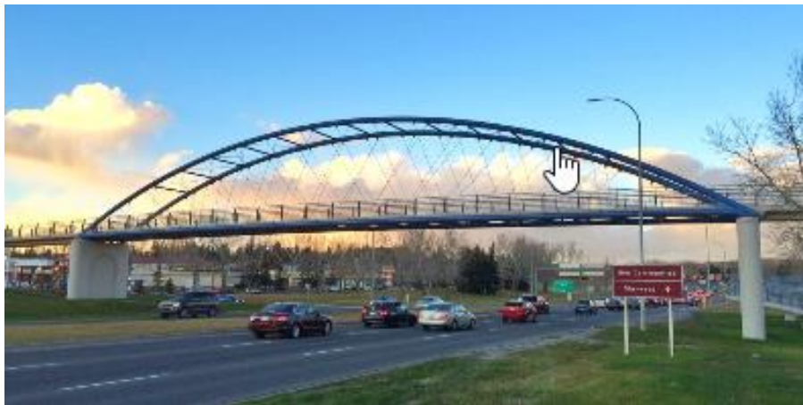
Figure 10: Network Arch Pedestrian Bridge Example
