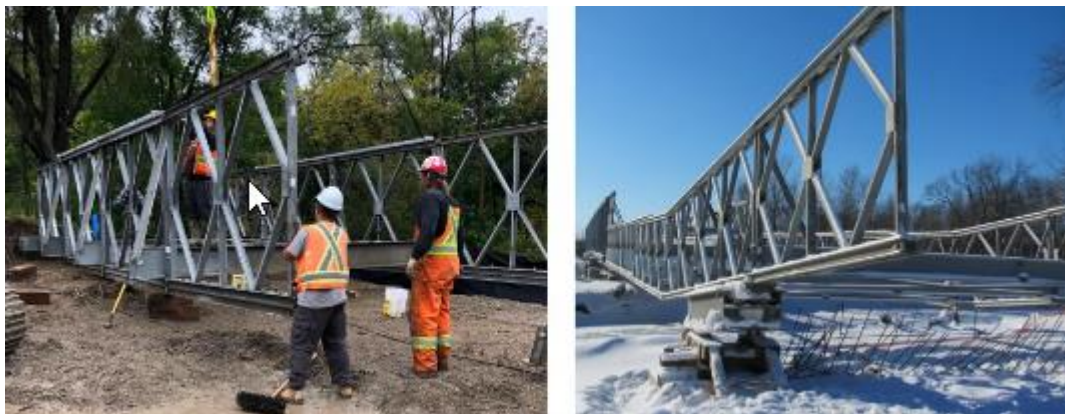
Figures 8 & 9: Assembly and Installation
