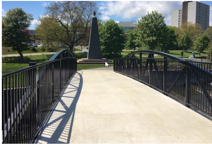
Figure 17: Bowstring Bridge Railing
