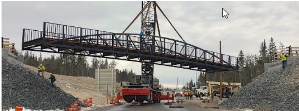
Figure 6: Installation of a Bowstring Truss Bridge
