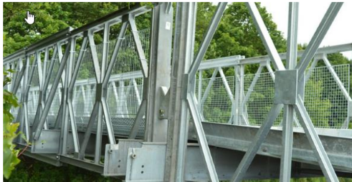
Figure 18: Modular Bridge Protective Screen System
